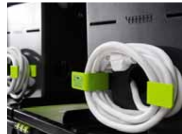
External cable management
