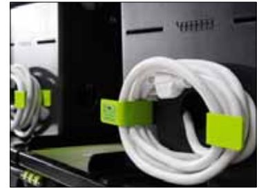
External cable management
